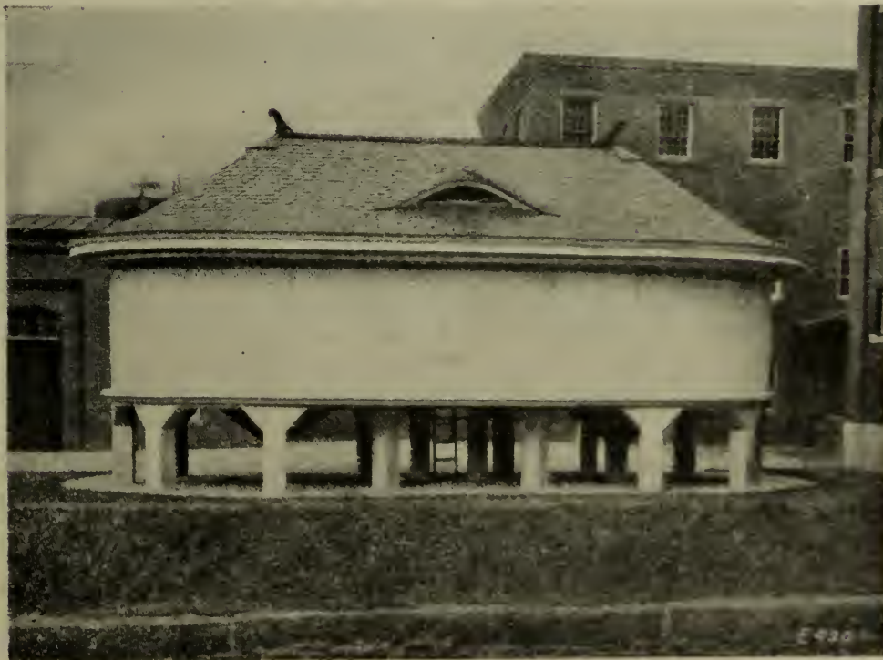
FIG. 5. CONCRETE TANK FOR CONTAINING SULPHURIC ACID.
